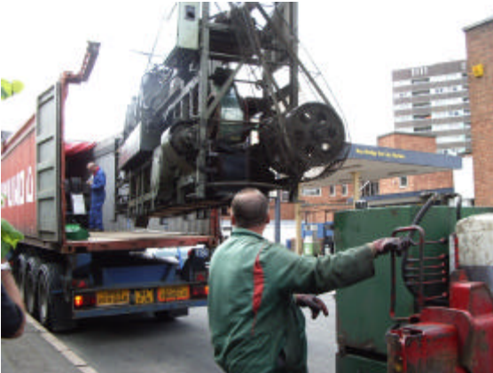
Removing the final machine
