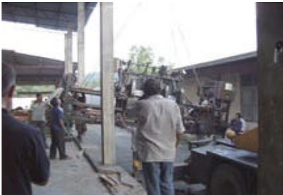
Unloading the machines at our factory.
